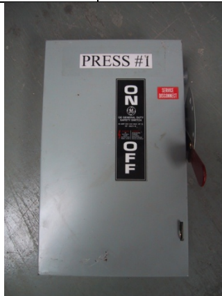
Electrical disconnects properly identified.
