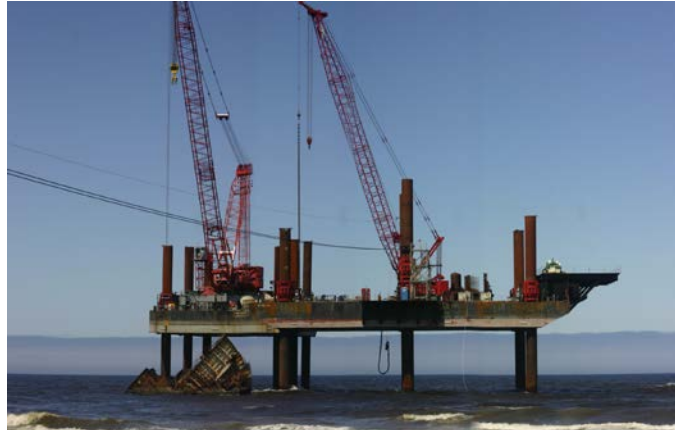
Barge with cranes held aloft on jacks.
