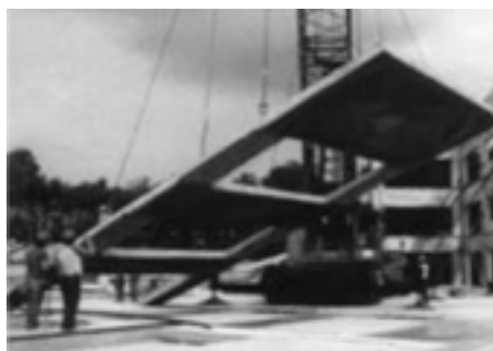
Contractors at the Home Depot site were largely unaware of tilt-up construction requirements.
