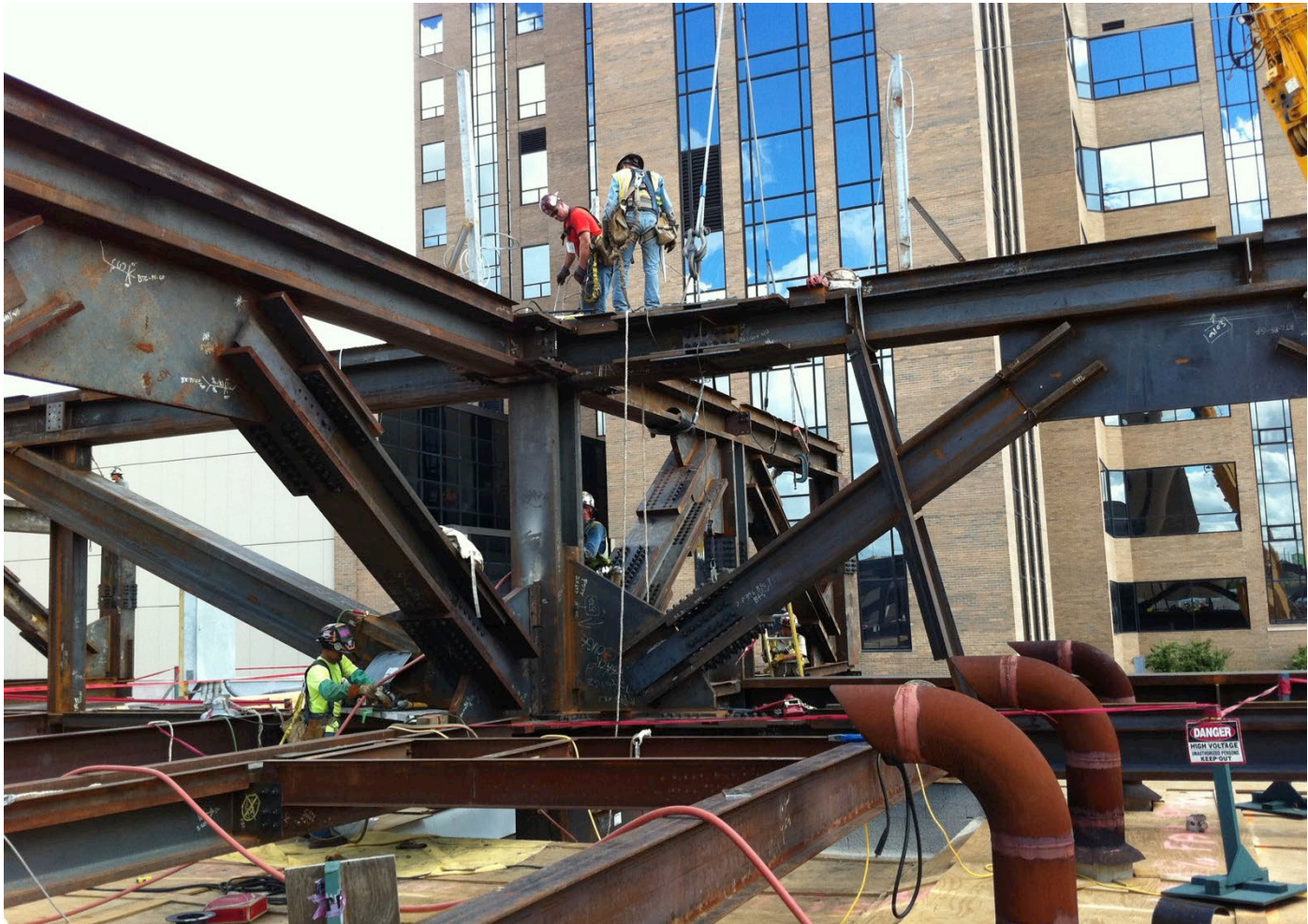
Truss Connection Pre-Heating
