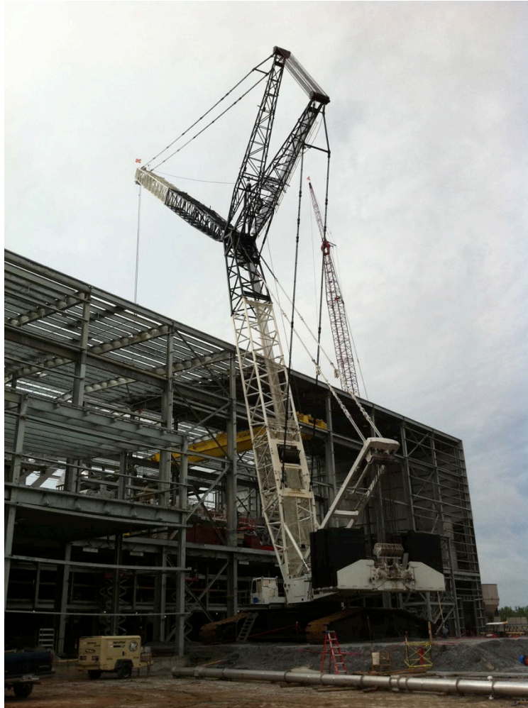
Steel Erection with Heavy Lift Crane
