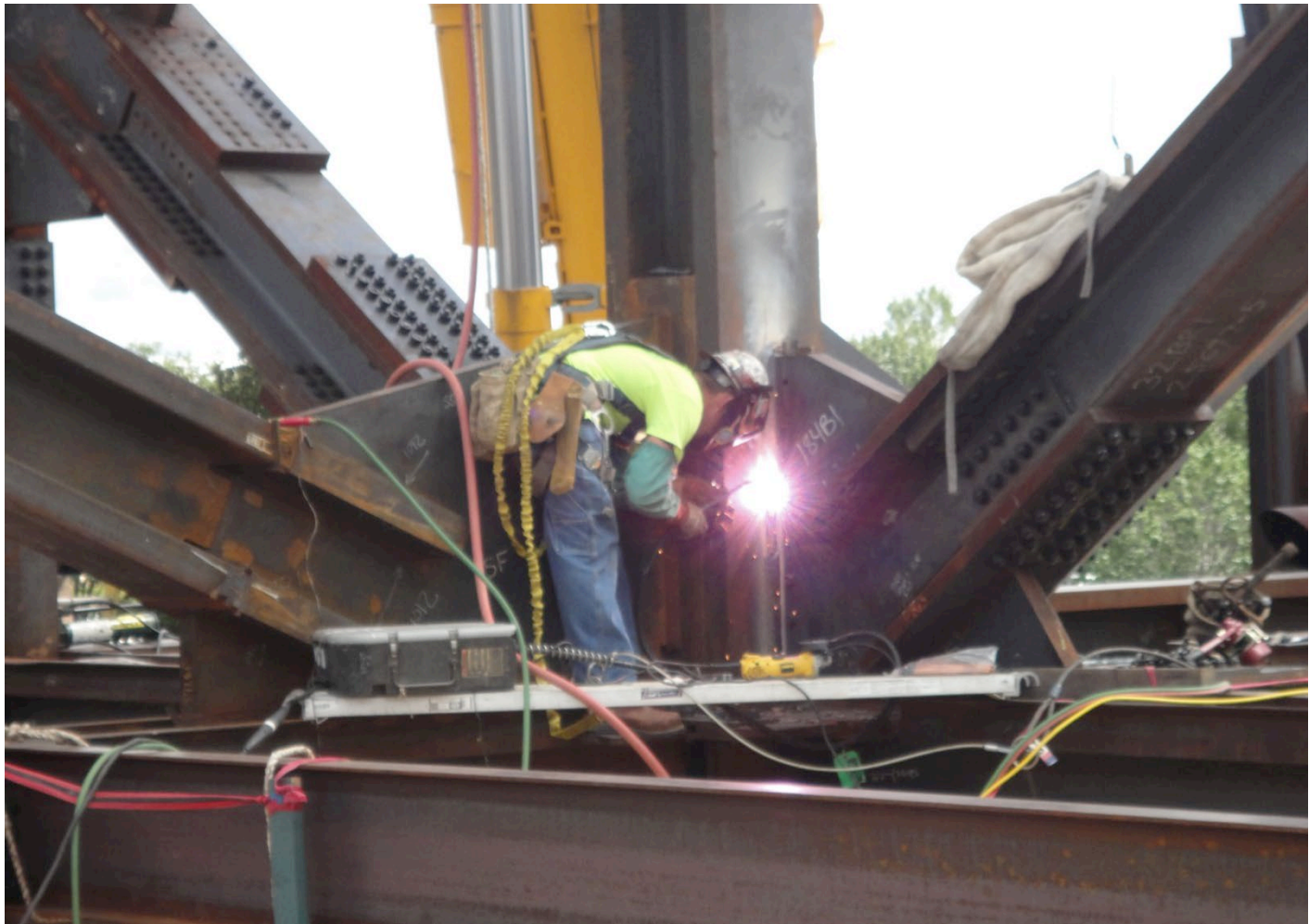
Welding Truss Connection
