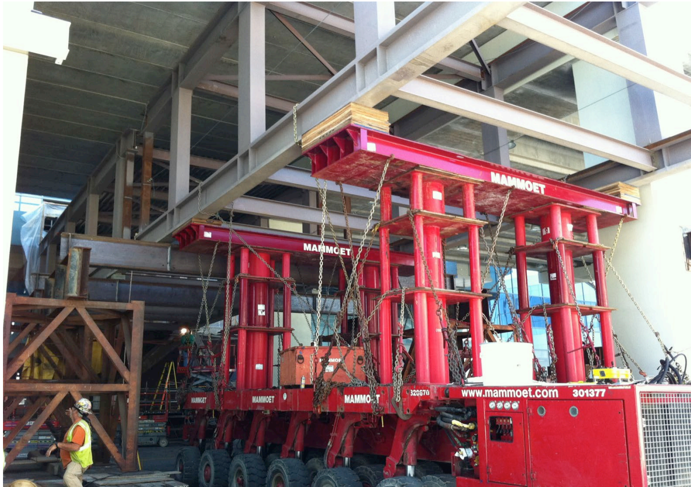
Truss Bridge Erection with Mammoet Transporter
