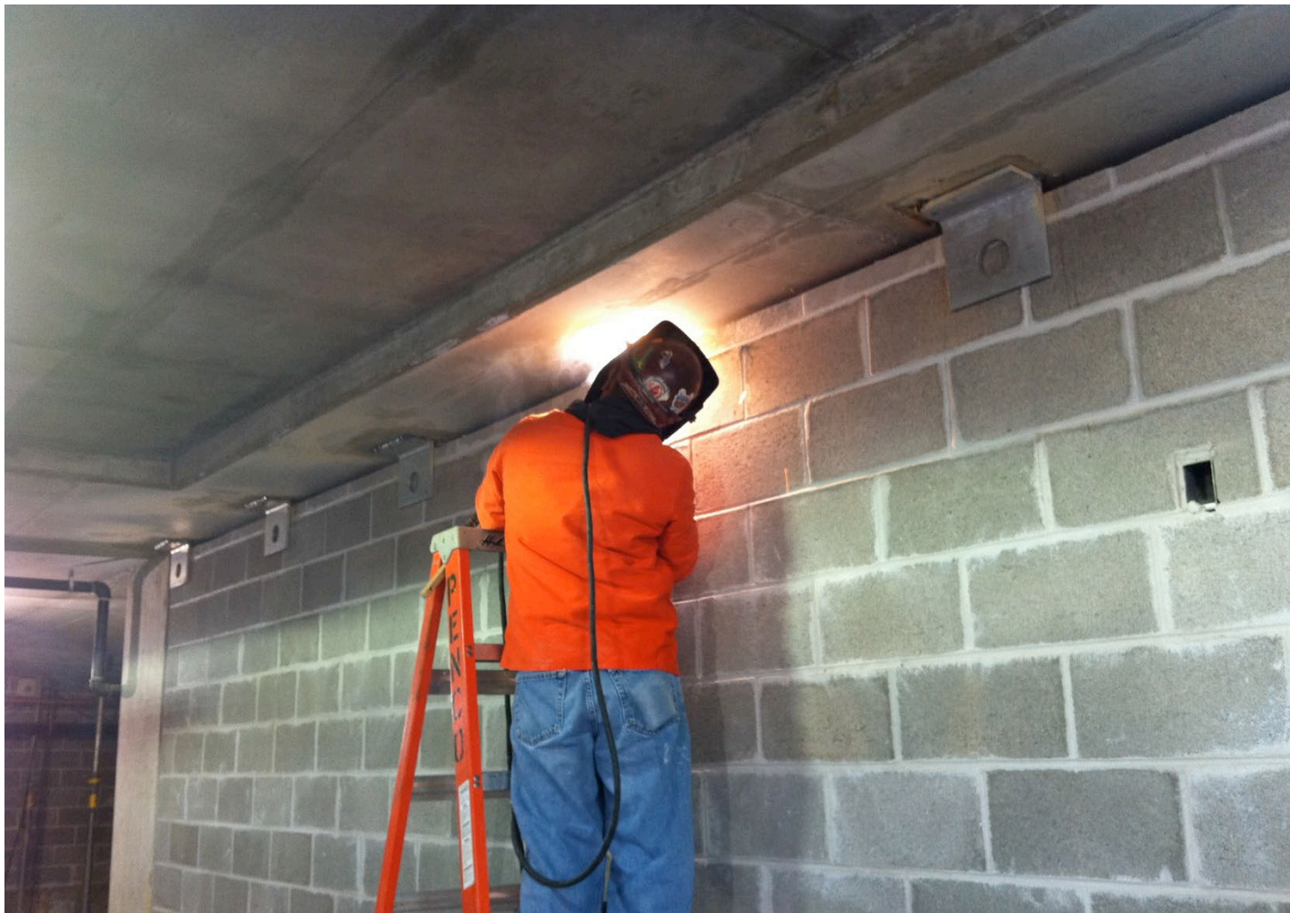
Welding Galvanized CMU Clips with Stick Welding with No Respirator
