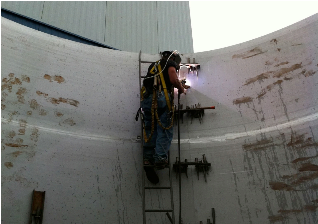
Stainless Vessel Welding
