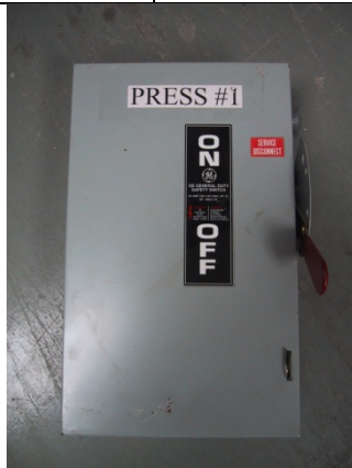
Electrical disconnects properly identified.
