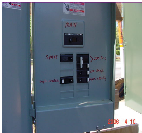
Electrical panel with all circuit breakers legibly marked.
