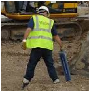
Instrument being used to locate underground electrical lines.
