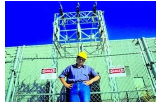
This exposed electrical equipment is guarded by an 8-foot fence.
