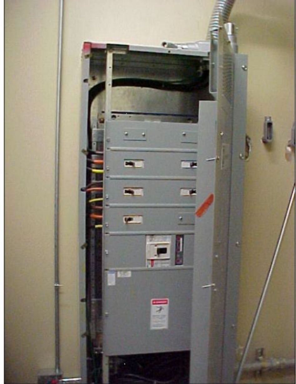
Door tied open to room with exposed live parts
