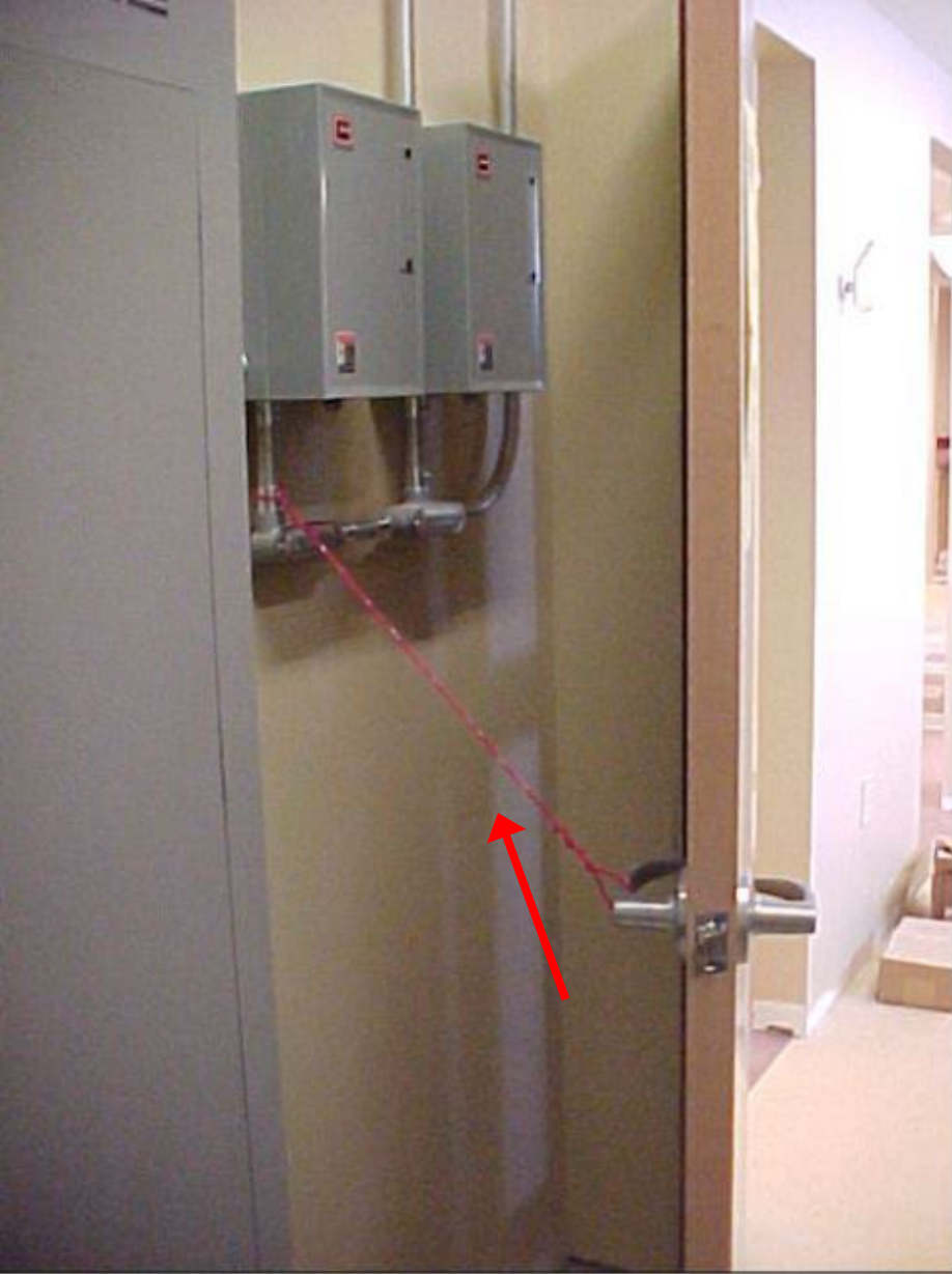
Door tied open to room with exposed live parts
