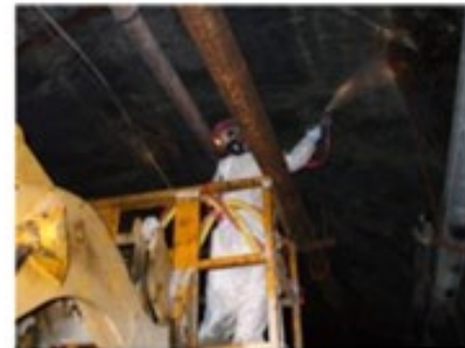
Underground mine wall consolidation
