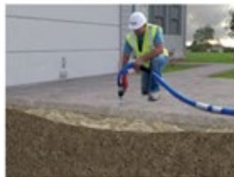
concrete lifting
