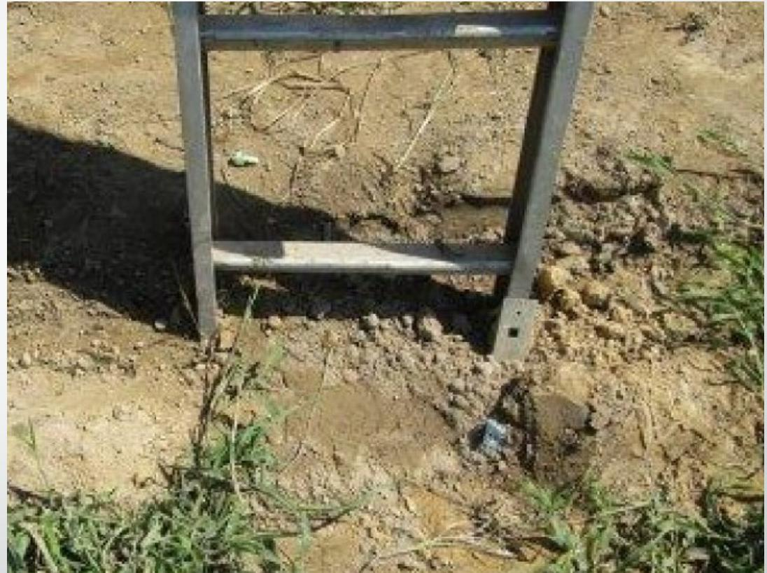
29 CFR 1926.1053(b)(16): Portable ladders with structural defects, such as, but not limited to, broken or missing rungs, cleats, or steps, broken or split rails, ....., were not either immediately marked in a manner that readily identifies them as defective
